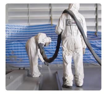
applications, providing the fastest back in service concrete coating available.
