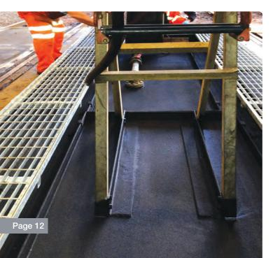
GLS 100R coatings are applied by our PTS trained technicians. GLS Coatings' mobile rigs include a spray machine, a portable generator and an aircompressor. Completing the kit is a collapsible spray-tent, with GRP mechanics. This ensures it complies with Network Rail's safety requirements.
